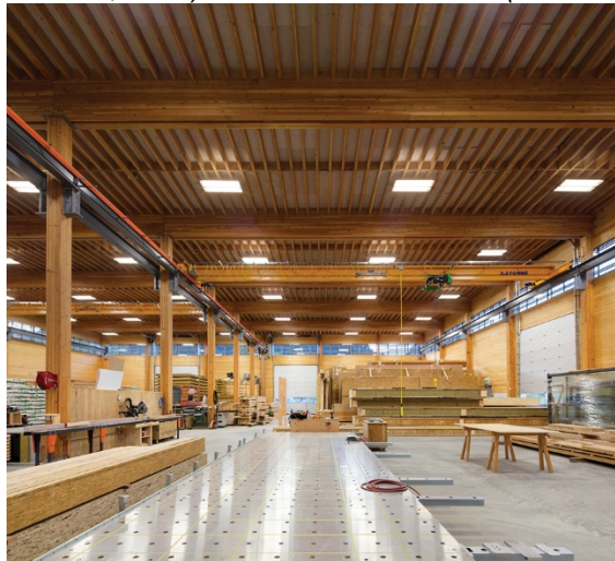
Figure 6 – Glulam Framing with CLT Wall Panels (Canadian Architect)
