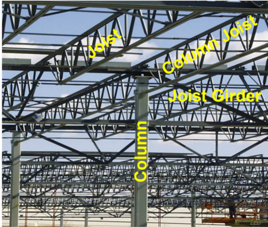
Figure 4: Truss System Including Truss Girders (Brothersen & Holtermann, 2018)
